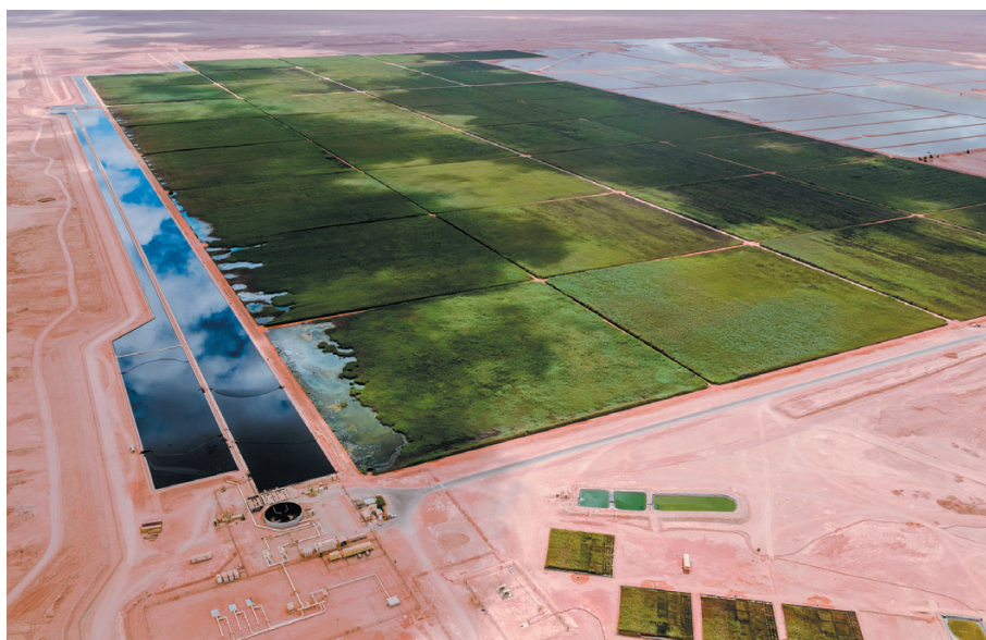
Natural reed bed water treatment project in Oman. Photograph courtesy of BAUER Nimir LLC. https://bauer.de/hr
